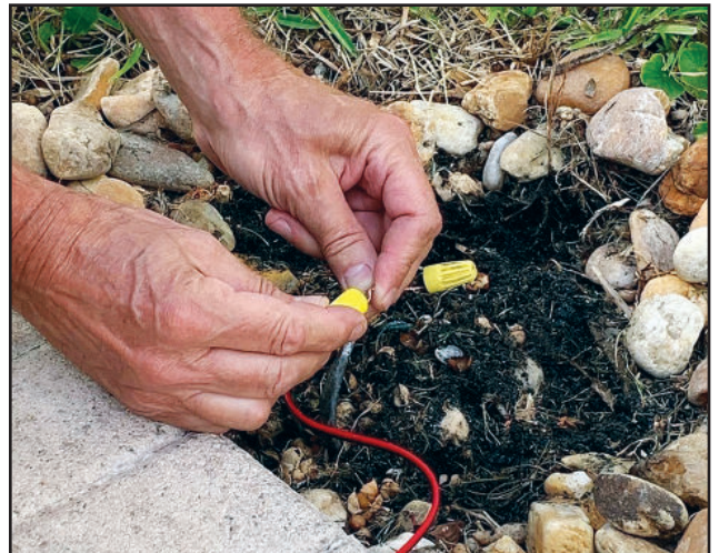
Attach the 2 wires from the Radiant Light to your new, or existing 12 to 15 volt, low voltage light system wire.
