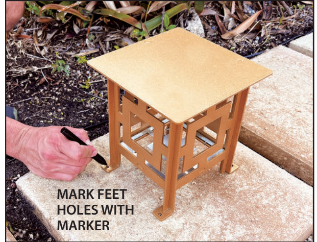
Mark feet holes with marker, don't forget to mark the hole for the low voltage wire to connect to the Lamp.
